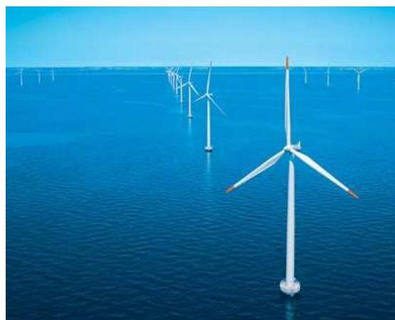
Figure 5.2: Offshore wind farm
