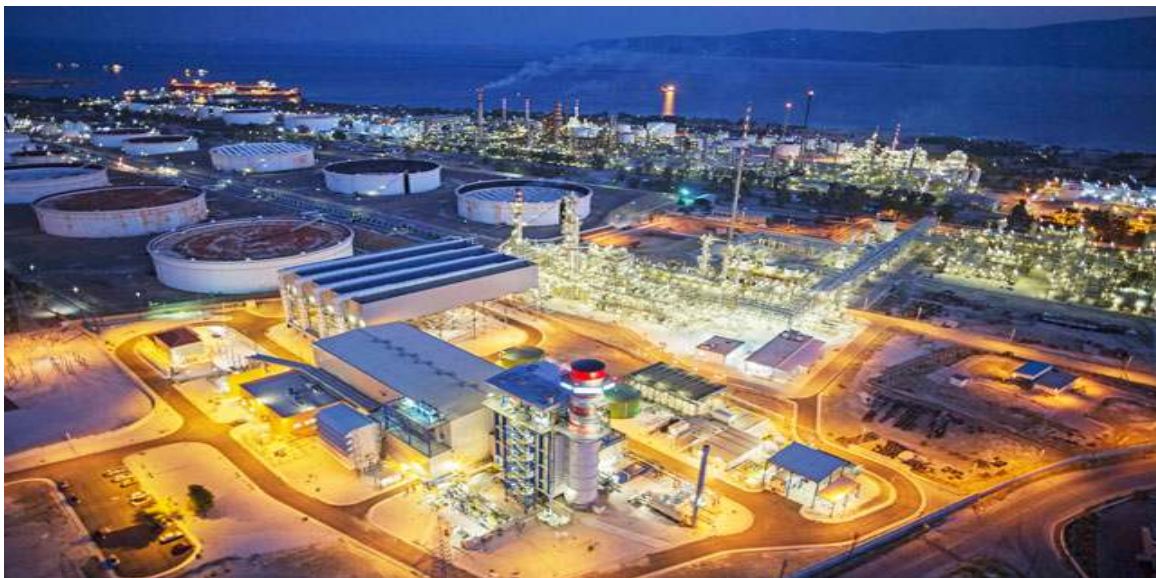
Figure 5.13: Motor Oil refinery in Agioi Theodoroi, Korinthos
