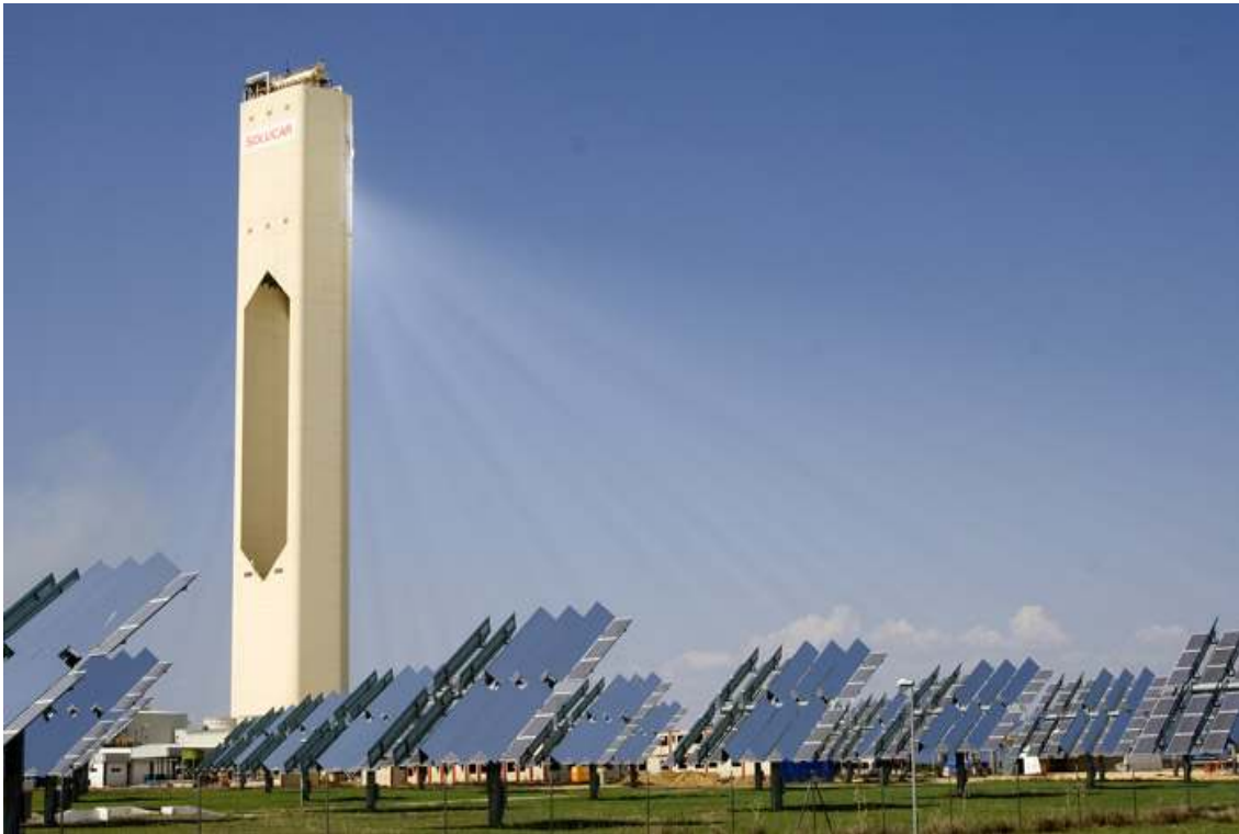
Figure 5.9: The CSP tower concentrates the light which is then utilized.
