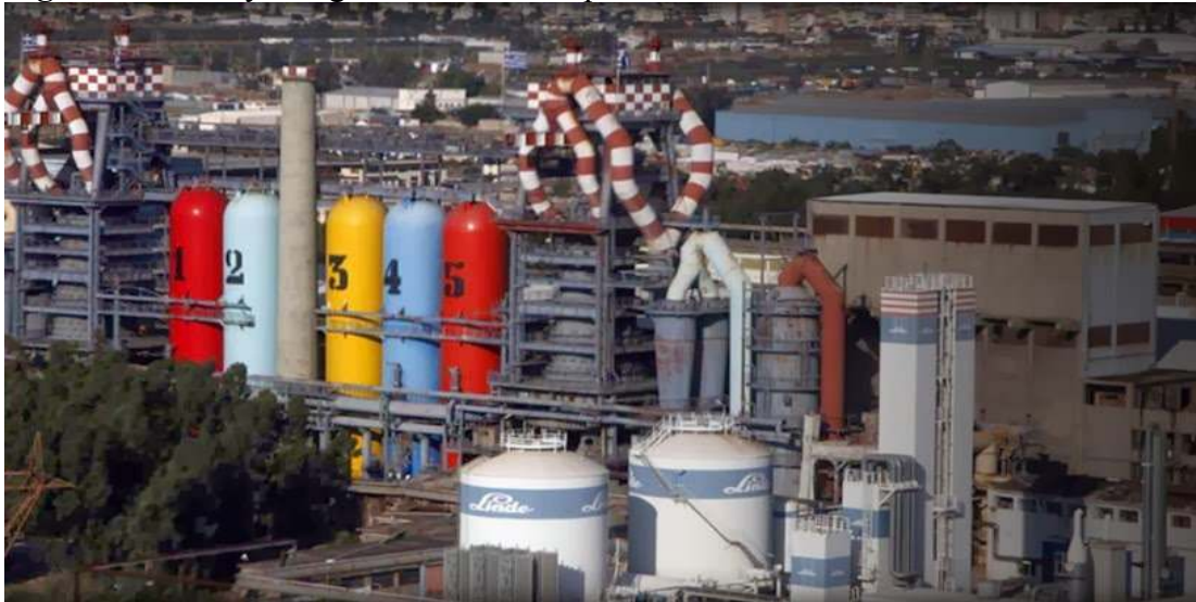
Figure 5.15: Halyvourgiki iron and steel plant in Elefsina.
